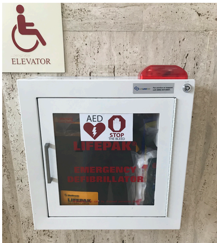
Figure 2. Image of Small (Public Access) Stop the Bleed Kit in Library AED Case
